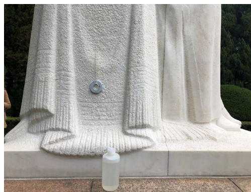
Figure 14. Water leaks from the sealed marble during water absorption test using Karsten's Test Tube. (Source: Tongji-ACL)
