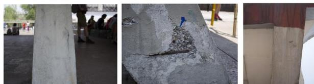
Figure 7. Exterior condition assessment. **Left:** exposed rebar reinforcement corrosion crack. **Center:** Concrete Spalling; **Right:** Moisture and Staining of Plaster (Pictures taken by Canadian students)
