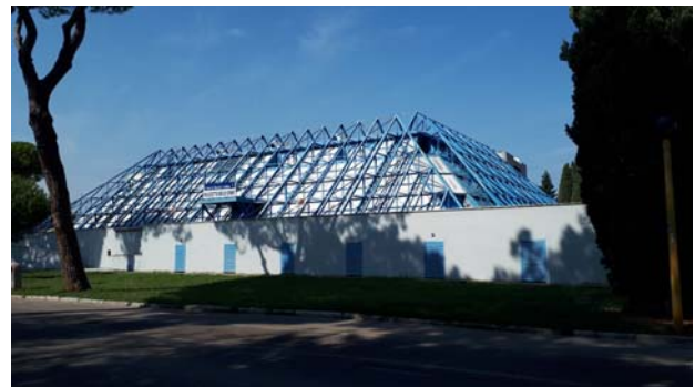
Figure 2. The current state of the Sports Hall built in 1983.
