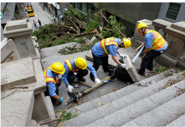
Figure 5: Towngas staff salvaging the broken cast iron column of the gas lamp.
