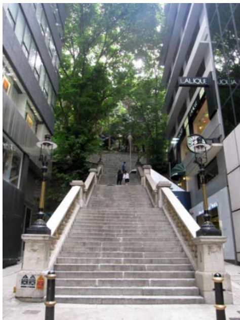
Figure 1: Duddell Street Steps and Gas Lamps, Central, Hong Kong before damage.
