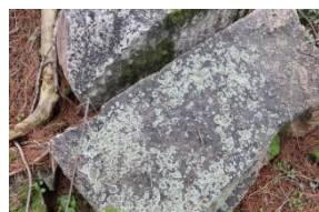
Figure.10-2 Weathering of stone in Shanjinxuan palace
