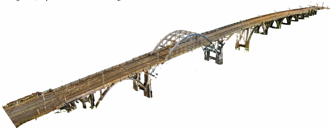
Figure 6. Registered point cloud of the whole bridge.
