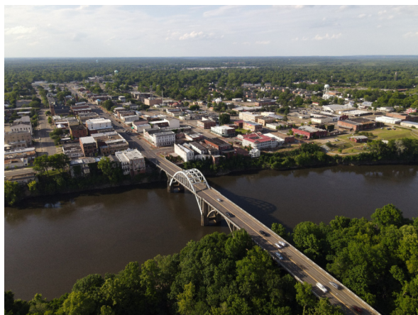
Figure 1. Aerial photograph of the Edmund Pettus Bridge.
