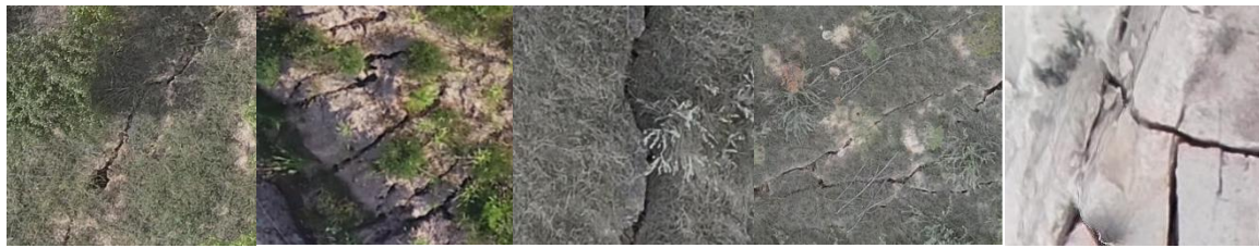
Figure 8. Examples of ground fissures in the study area.
