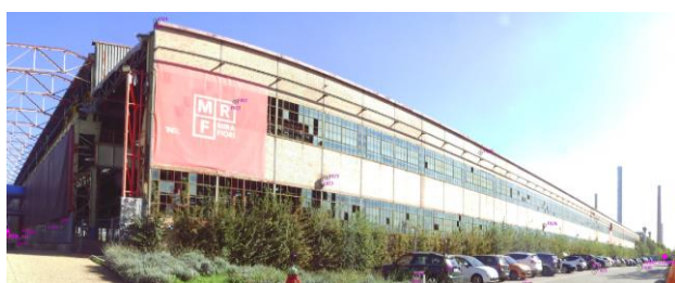
Figure 2. Image from Terrestrial Laser Scanner (TLS) camera.
