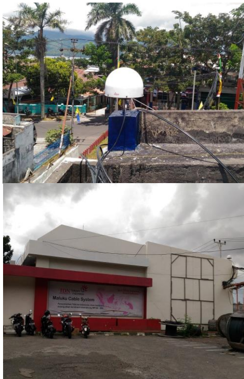
Figure 3. Geodetic Control (CORS) at Telkom office
