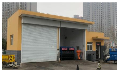
Figure 5. Missing refuse collection stations at both point and surface levels.
