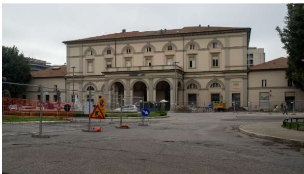
Figure 1. Current state of the Fontivegge station affected by requalification works.
