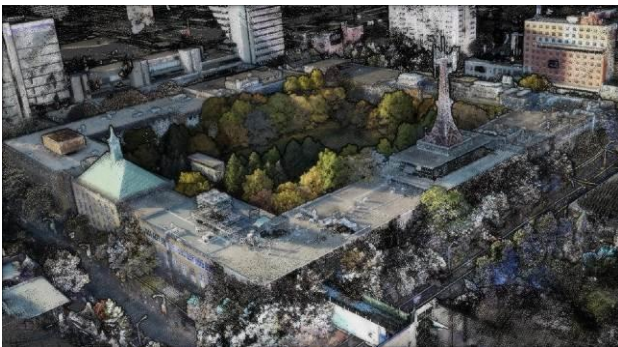
Figure 13. Present occlusion on the combined dataset on one of the building's facades due to tree coverage.
