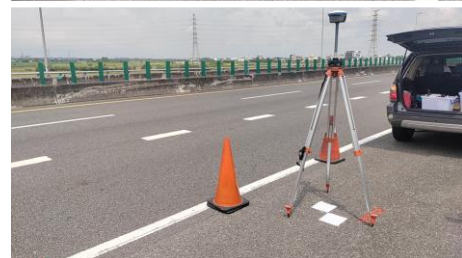
Figure 7. Ground control points surveying by e-GNSS (on the expressway, yellow triangle).
