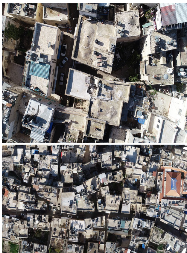
Figure 5. Preliminary images of the detection process. Above, raw image from drone with integrated location metadata thanks to the GPS systems of the aircraft used. Chunks for SfM photogrammetry were made for urban districts and georeferenced according to GPS targets. Object detection training took place on the raw images, and recognition and identification was initiated on the orthoimages to make the object georeferencing processes effective. This process also makes it possible to develop systems of scheduled surface inspections, planned over time.
