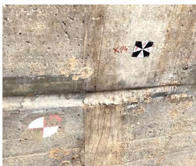
Figure 3. Markings sprayed (bottom-left) and glued (top-right) on the hydropower dam.
