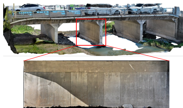
Figure 2. Facade Orthomosaic of a Pier from the Jujeong Bridge
