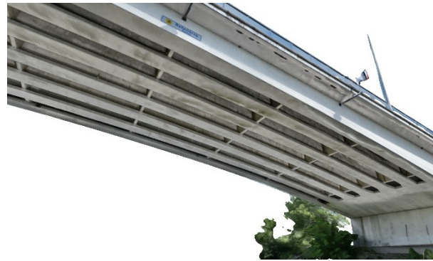
Fig. 7: Highly detailed photogrammetric model with high coverage in difficult to reach areas
