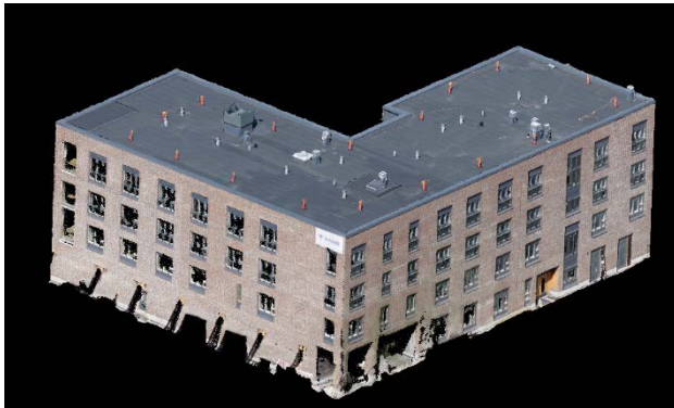
Figure 2. The colored dense 3D point cloud of the test building.
