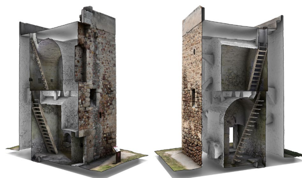
Figure 2. The high-fidelity master model of Torre del Mar. The textured polygonal mesh integrates the exterior envelope and interior spaces, serving the multimodal XR ecosystem. (Modelling and editing: E. Pupi)
