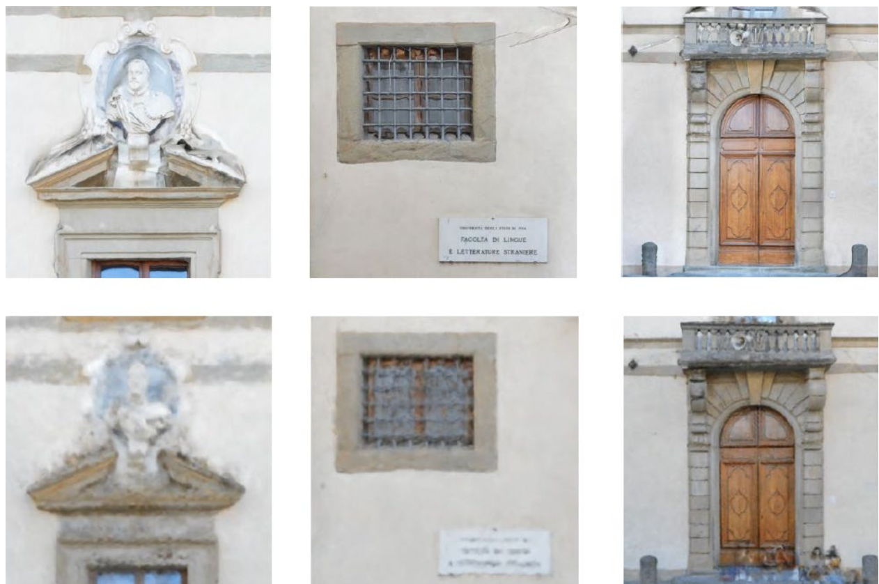
Figure 10. Façade of Palazzo Boileau. Details of the photogrammetric mesh (above) and the volumetric rendering generated by the NeRF (below).
