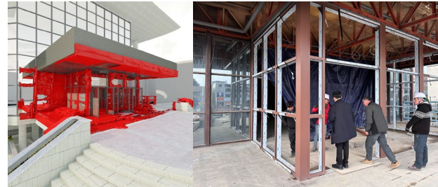
Figure 7. LiDAR point cloud data overlays to planning model for revising main gate design as reference of the original (left, source: KLIMA architects); The construction site (right)
