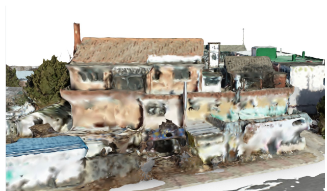
Figure 11. It shows the appearance of the building in the raw mesh model.
