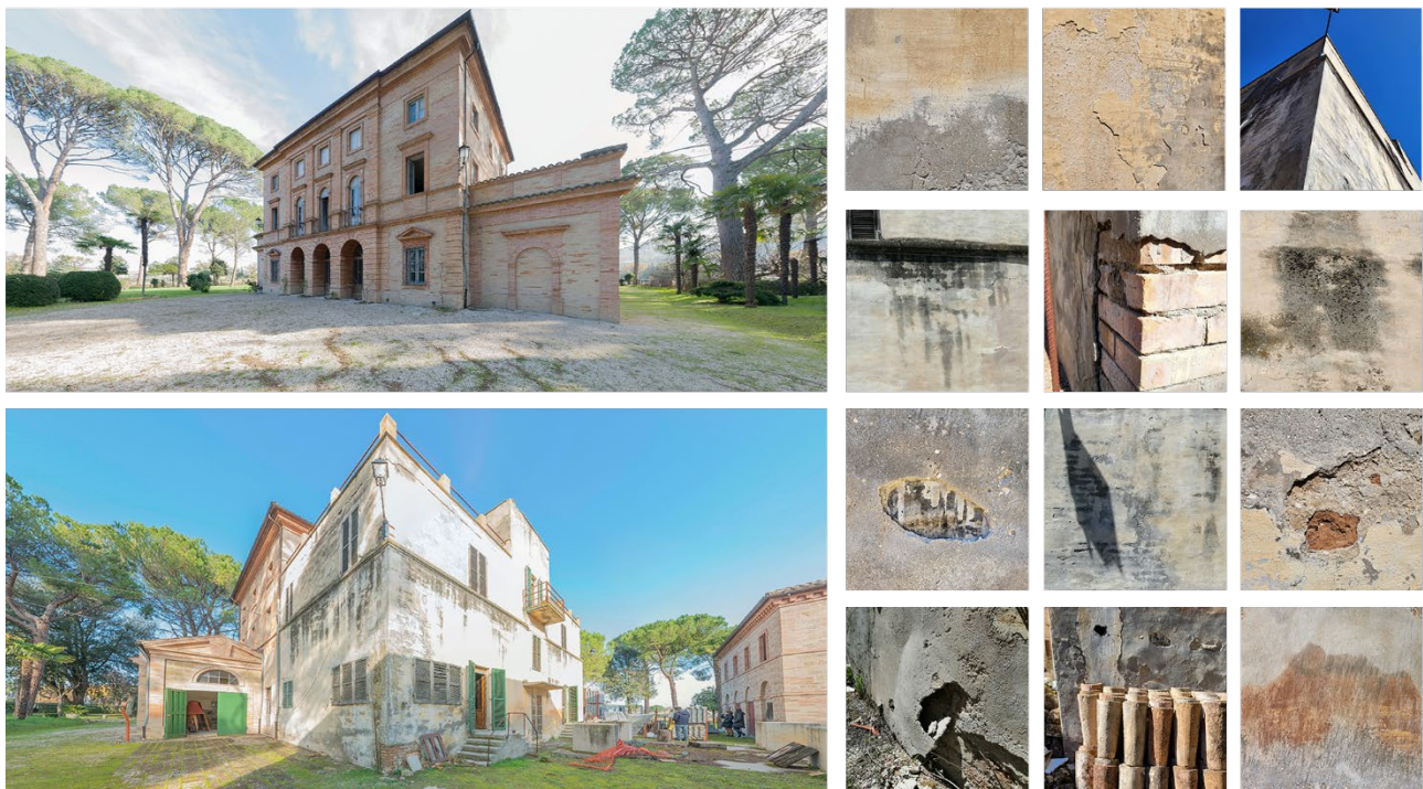
Figure 1 Villa Leonardi, Treia (MC), Italy. General views of the exterior and details of some alteration/decay phenomena.
