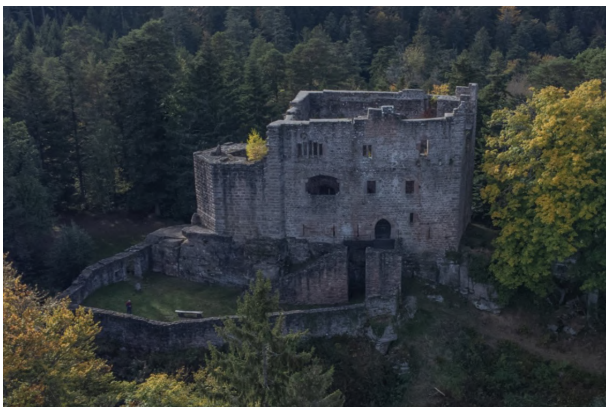
Figure 6. Front view of the Birkenfels Castle
