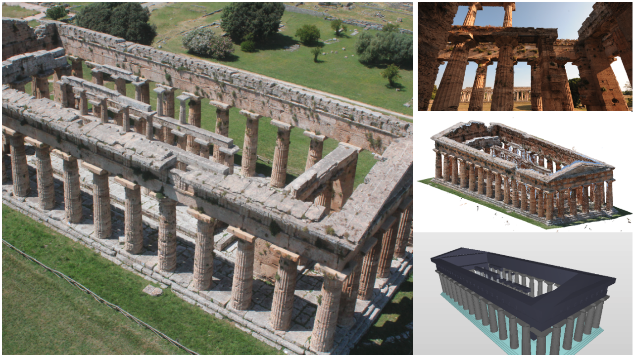
Figure 1: Overview of the project inputs: (left) hand-held and UAV images, point clouds and BIM model.
