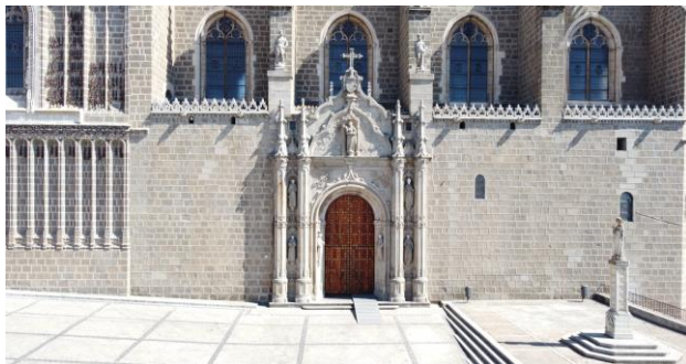
Figure 5. View of the main entrance elevation to the Monastery of San Juan de Los Reyes.
