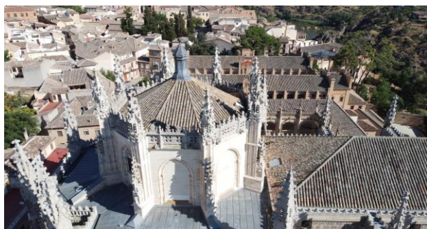
Figure 1. Drone view of the cloister and roofs of the Monastery of San Juan de Los Reyes.
