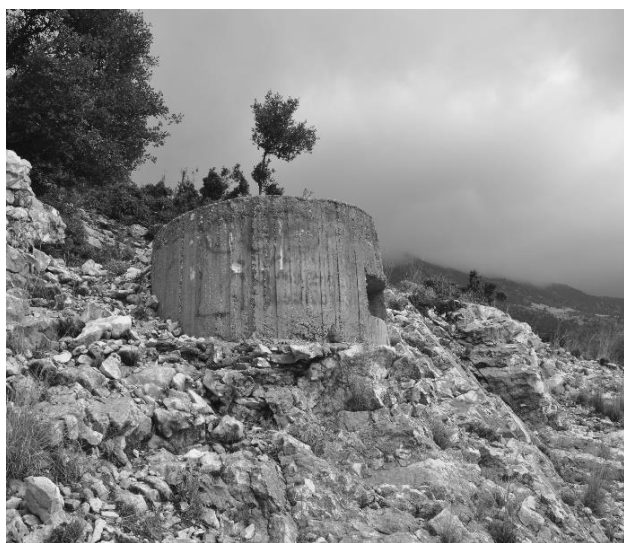
Figure 2. XS-type bunkers. State of the art view
