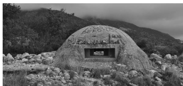
Figure 4. Bunker type S. Survey and view of the state of the art
