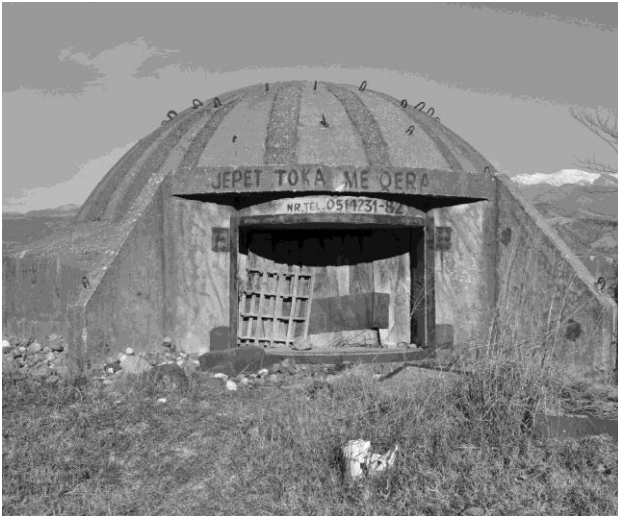
Figure 8. Type M bunkers State of the art view
