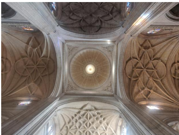
Figure 2. Segovia, the Cathedral, view of the intrados of the internal vaults.
