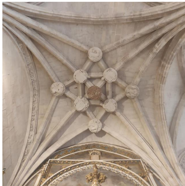
Figure 11. Detail of the vaulted system of the cloister of Segovia Cathedral.
