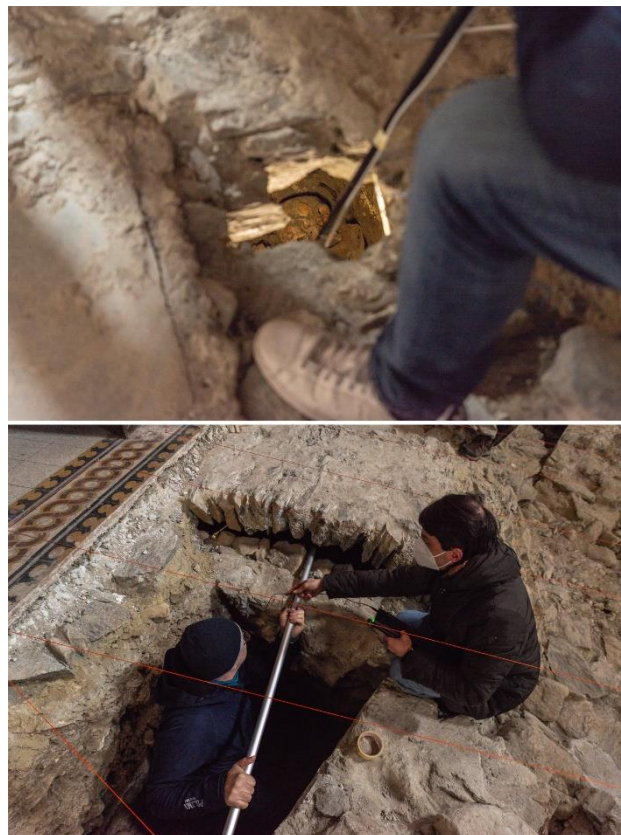
Figure 4. Insertion of the 360° borescope in the two breaches.
