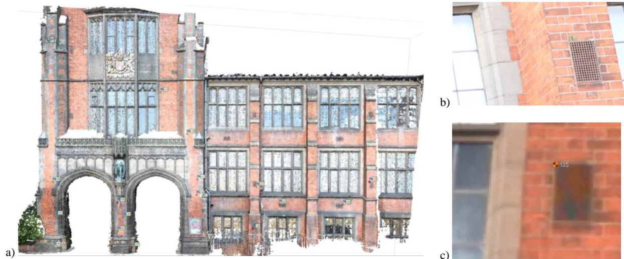
Figure 2. (a) Test field target distribution on the façade of The Arches (Newcastle University campus), illustrated with a dense point cloud generated using Canon SLR imagery. Imagery of the façade captured by the (b) Canon and (c) GS18i over GCP 125, located at the corner of an air brick.
