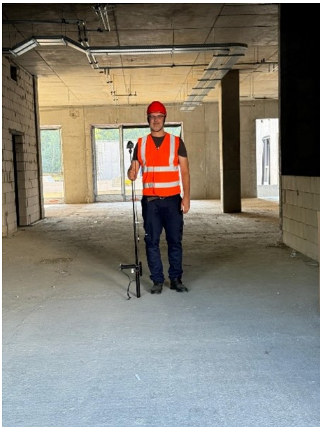
Figure 5. Configuration 5: Construction site survey with device on the long stick.
