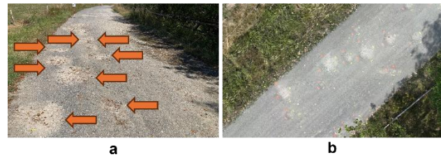
Figure 2. (a) Defects of varying severity as seen from the ground; (b) defects as seen from aerial imagery collected via UAV (Unmanned Aerial Vehicle) photogrammetry, after marking with fluorescent paint.
