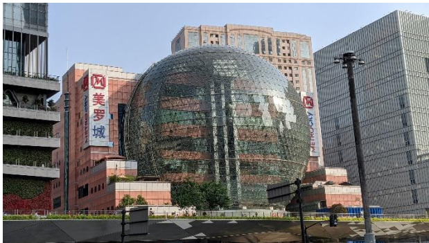
Figure 1. Demonstration of the Meiluo Cheng experiment building.
