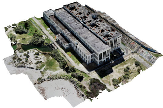
Figure 6. Output from OpenDroneMap processing of aerial images of Fremantle power station
