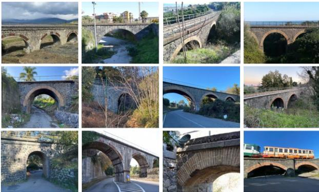
Figure 5. Some bridges of Circumetnea. Note, in particular, that they are heterogeneous in terms of materials, geometry, and number of arches.
