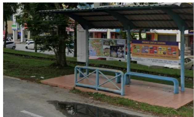
Figure 14. Bus Stop at Bandar Saujana
