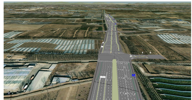
Figure 4. Road maintenance scene.
