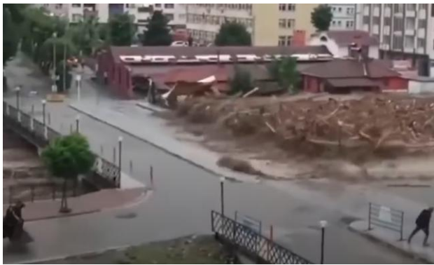
Figure 8. Debris blockage of main vehicle bridge.
