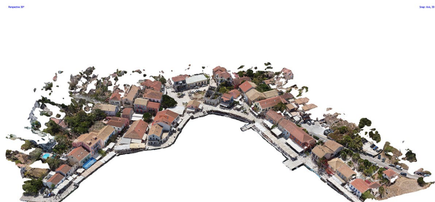
Figure 17. Fiskardo Port, dense point cloud, as seen from the dock.
