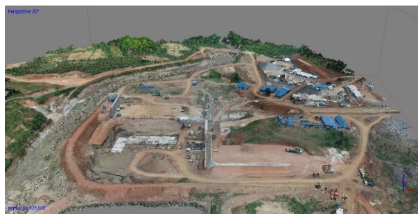
Figure 5: Illustrates the as-built data
