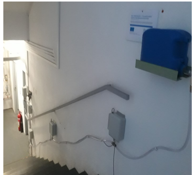
Figure 5. Configuration of the hydrostatic sensors in the real testing object.
