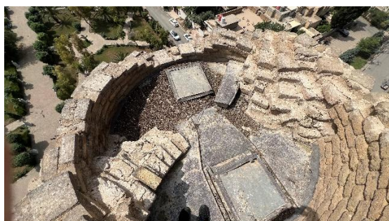
Figure 14: The moisture clearly visible at the base of the minaret (left up), a very good condition of minaret part, no cracks are visible
