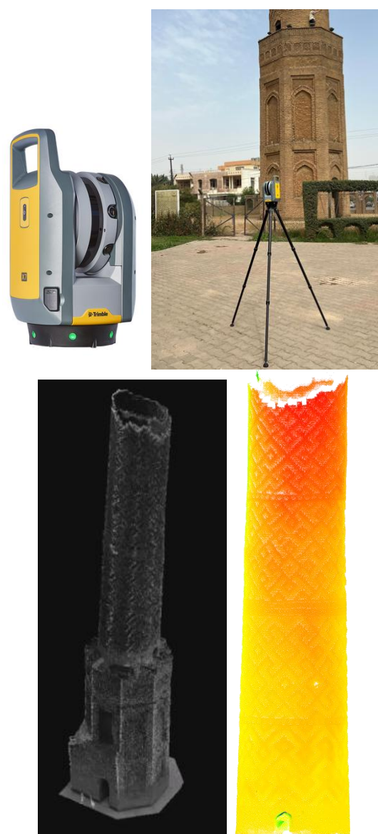
Figure 5: Used laser scanner Trimble X7, (upper part), point cloud from measurement, photo from one of 67 scanner position (left) and deformation of the upper part of minaret (right)
