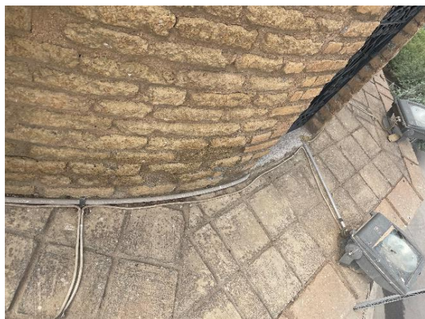
Figure 14: The moisture clearly visible at the base of the minaret (left up), a very good condition of minaret part, no cracks are visible
