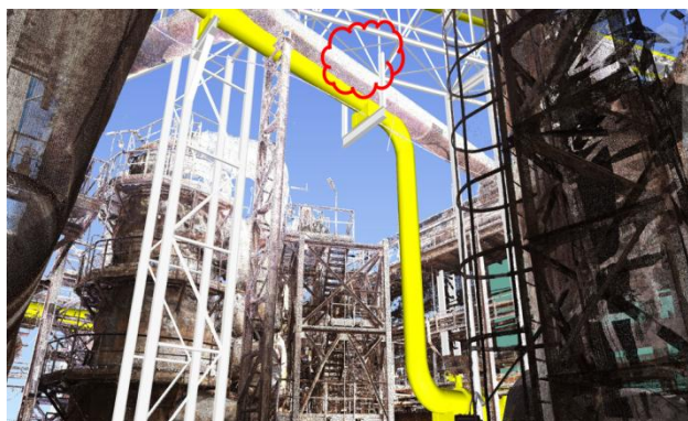
Fig. 13. Fragment of a detected clash based on the comparison between the actual point cloud and the design model.
