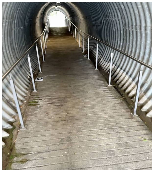
Figure 2. Tunnel in Préverenges. Narrow, dark, high contrast, and big differences in scale make photogrammetric processing very challenging.
