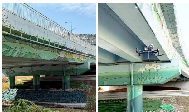
(a) A bridge located in Shenzhen (b) The UAV under the bridge
