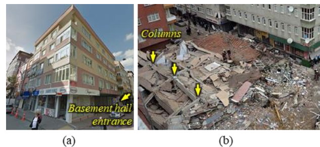
Figure 5. Investigated building: (a) before collapse and, (b) after collapse (Modified from Google, 2022; IHA, 2016)
