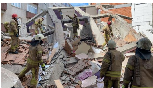
Figure 9. The collapsed building (Web-4)
