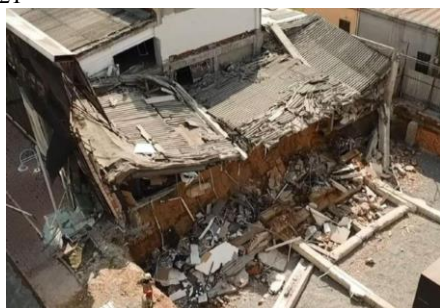
Figure 4. A picture of the collapsed building (source: DHA, from evrensel.net)
