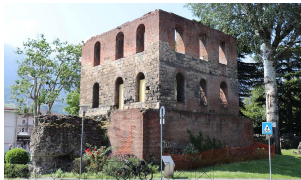
Figure 1: The building selected for the practical simulation inside the training activity, Tour De Pailleron, Aosta, north-west view.
