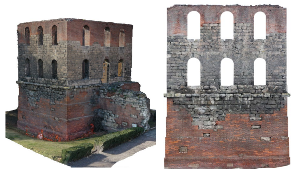
Figure 3: the survey results of the Tour De Pailleron: laser scanner point cloud (top), photogrammetric mesh model (bottom-left), orthophotos (bottom-right)
