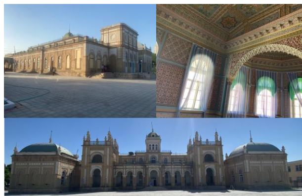
Figure 1. Photos of outdoor and indoor of Emir Palace.
