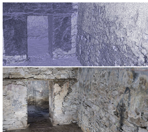
Figure 6. Interior View in the Naos of the Model (top: Wireframe; bottom: Textured Mesh).
