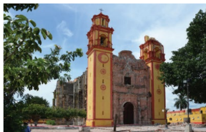
Figure 2. Typical damage of facade and bell towers – Historical Churches September 2017 Puebla, Mexico
